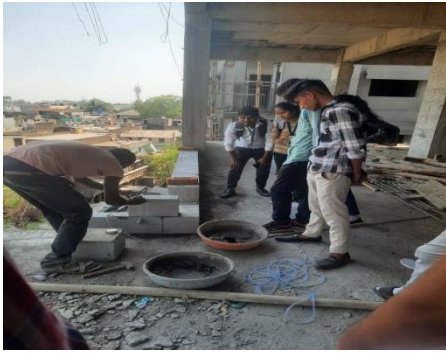
ACC block Masonry Work
