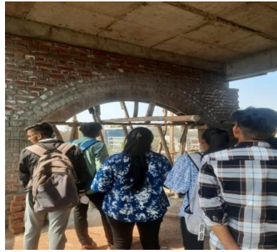
Ongoing Arch Work
